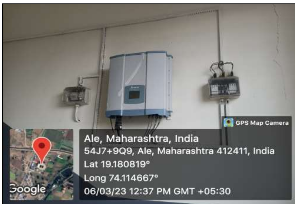
Installation of Solar System
